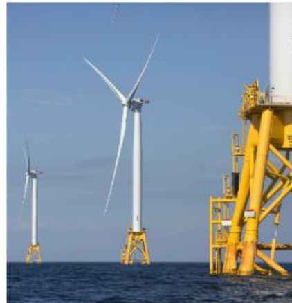
Offshore wind turbines near Block Island, R.I. A large offshore wind energy project planned off the coast of New Jersey will connect onshore to two former power plants, and cables will run under two of the state's most popular beaches. Michael Dwyer / Associated Press, File
